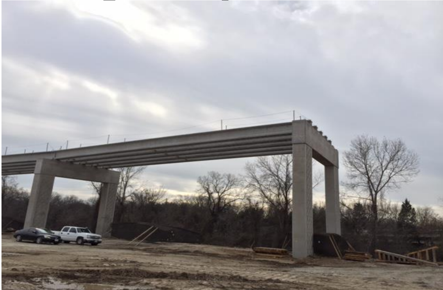
Southbound IH 45 to Southbound CF Hawn
