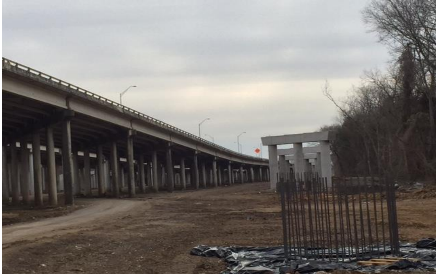
Bridge Work – Pennsylvania to Southbound IH 45 Bridge
