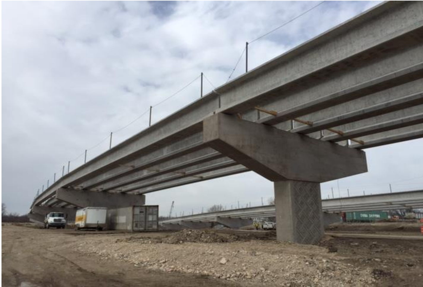
Beams set on IH 45 to Lamar
